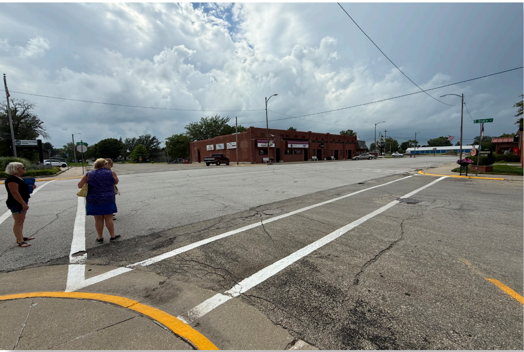
The existing crosswalk is 60 feet across. Shown below are proposed bump-outs that reduce the crossing width to 35 feet.
